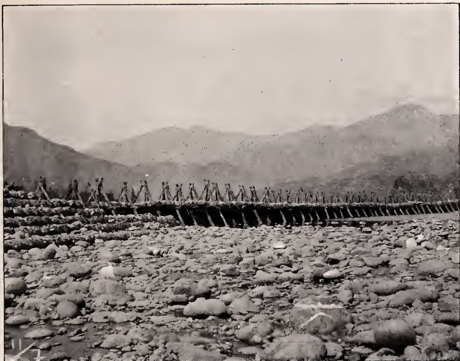
Near view of 'barrage' in position, shutting out the water from one of the two channels into which the river is here divided.
